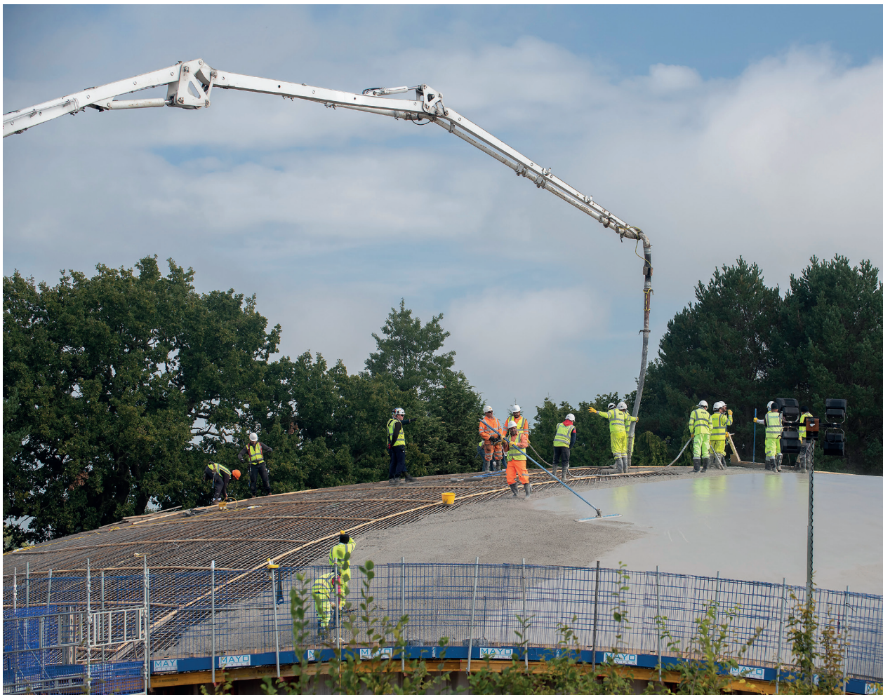
Left and top: The main structure of the First Light Pavilion is an in situ concrete dome which was then buried beneath earth and seeded to appear as a “hill” in the arboretum of the observatory. The dome was cast in one go, starting by the entrance to the south. The pour took 10 hours
