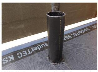
Install the underlayer, ensuring that it laps with the AVCL and provides a watertight seal to the soil vent pipe.
