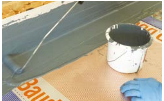
No.4: Reinforced LiquiDETAIL is applied to all upstands and details.
