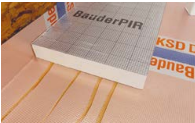
No.2: Bauder insulation installed with insulation adhesive.
