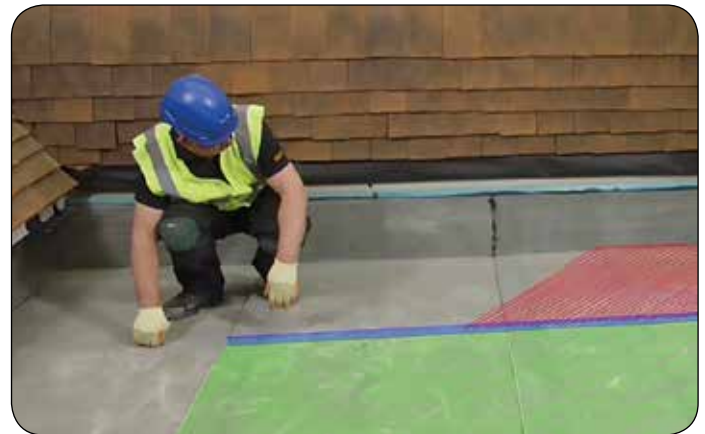
Torch-free insulated upstands to existing low eaves
