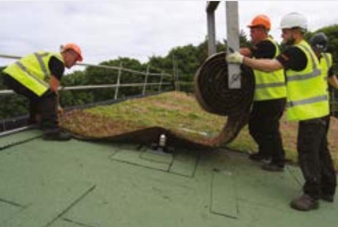
Long length rolls are used to speed up installation process.
