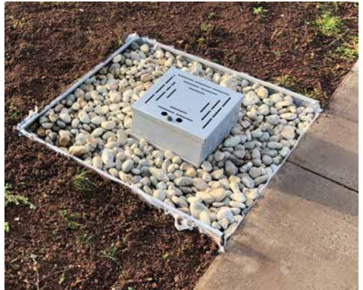
BauderBLUE ALU250 inspection chamber. As the total build-up of the blue-green roof system was over 200mm, a 100mm height adaptor was added to ensure the top of the chamber was level with the surrounding landscaping. The barrier between the outlet and the vegetation comprises of 20-40mm rounded pebbles. This will prevent unwanted growth obstructing the drainage system.
