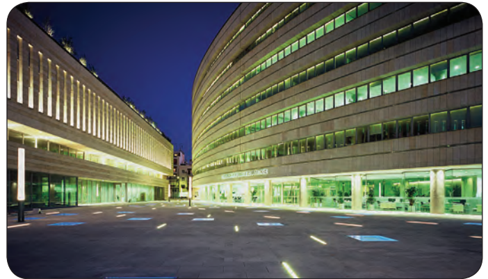
DPH Pedestals supporting large format marble slabs
