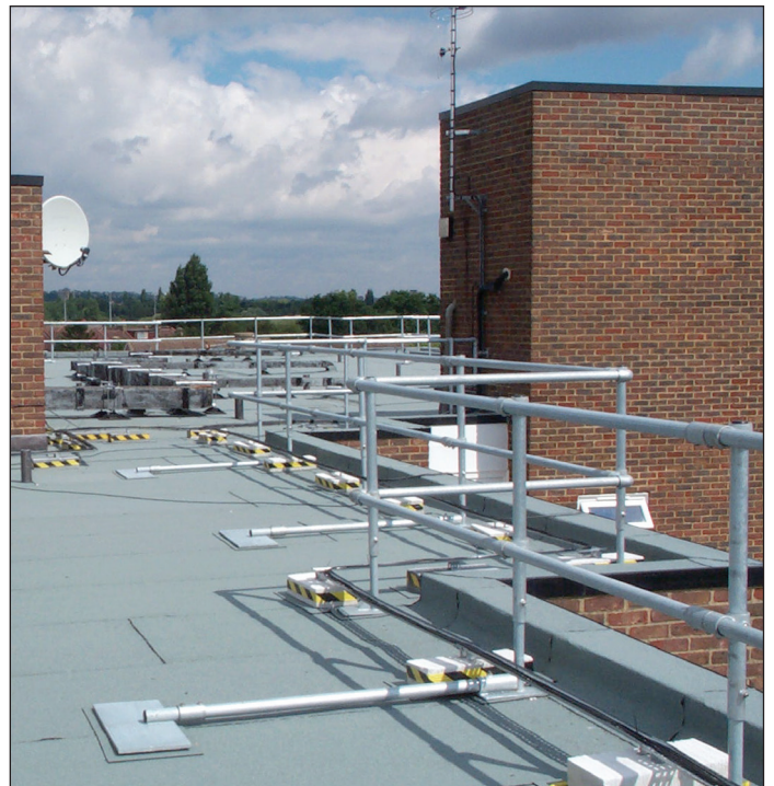
▲ Edge protection provided by free-standing handrail system
