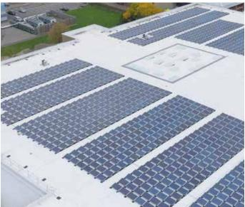
A flat roof is the ideal place for a solar PV installation as it provides an unobstructed space that is perfectly positioned to catch as much sunlight as possible.
