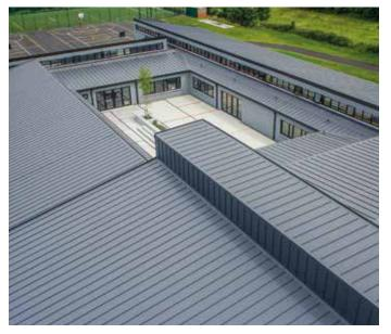
A single ply system provides many advantages to the modern building, particularly if weight and load bearing limits are an important consideration.
