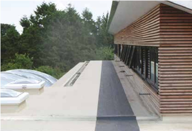
Thurlton Primary School, Norfolk (embossed walkway membrane with Thermoplan T installed in harmony with bituminous membrane)
