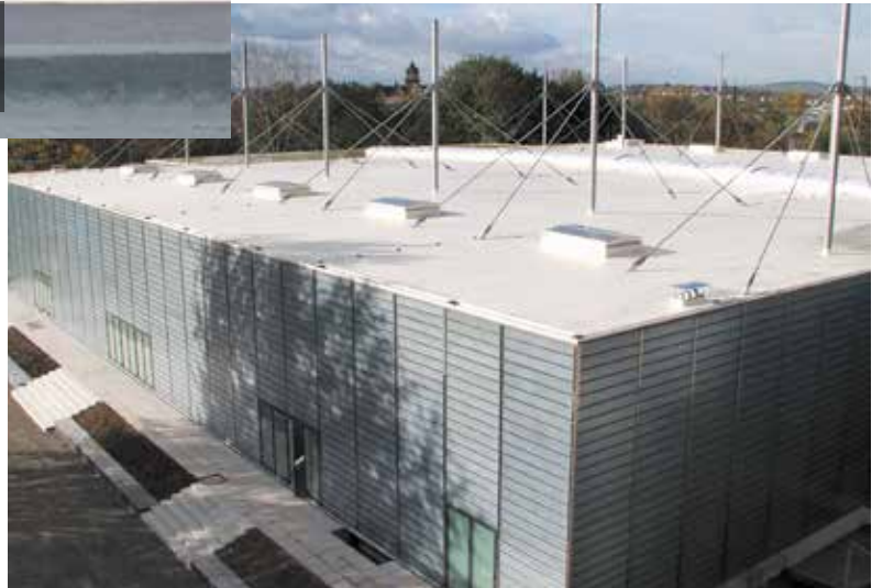
Thurlton Primary School, Norfolk (embossed walkway membrane with Thermoplan T installed in harmony with bituminous membrane)
