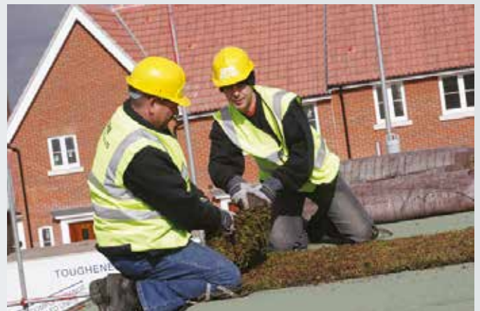
Short 2m rolls of XF301 Sedum System installed by hand.
