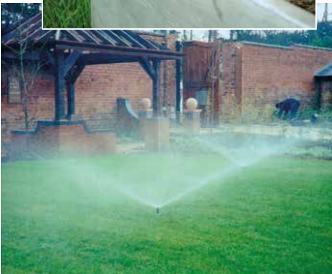
▲ Perforated pipe irrigation installed within a raised brick built planter
