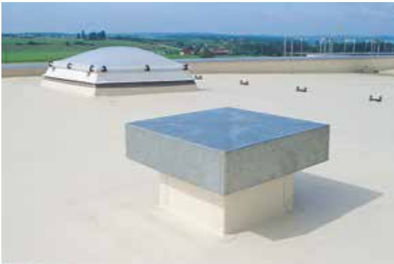
Thurlton Primary School, Norfolk (embossed walkway membrane with Thermoplan T installed in harmony with bituminous membrane)
