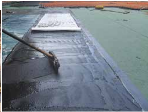
Hot Melt being installed
