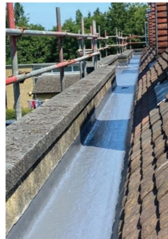
The 100m perimeter gutter with a new Bauder liquid waterproofing overlay.
